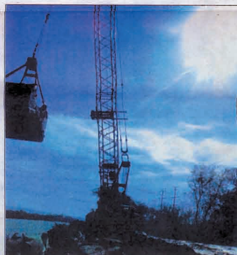
Al Rivers utilizes the power the 3900 W 115 ton Liebherr Crane to remove silt that's been loaded into a hopper (silt that is removed from the canal bottom is then transferred, via hoppers and cranes, to the silt pond).
