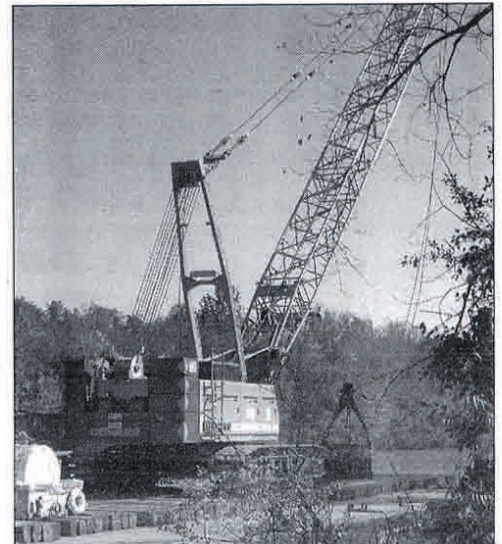
Liebherr 115 ton crane on one of the barges removes silt from the canal bottom which is then loaded into a scow to be taken to the UDS.
