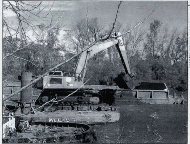
The Hitachi EX 750 track hoe removes silt and sand from the Canal bottom and transfers it to the scow. The scow is then taken to the UDS where crane operators transfer the silt to the UDS.
