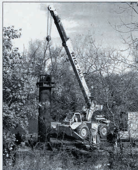
Spuds are lifted on one of the barges with a Rig-All Crane to adjust the barge's positioning.
