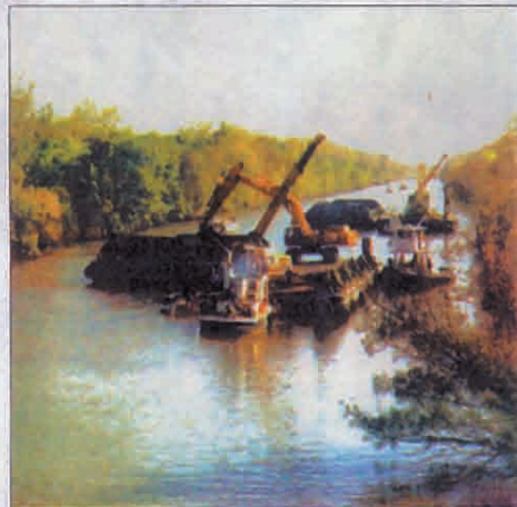
Recreational boats can be seen in the background of the dredging operation at the Erie Canal in Utica, New York. Cranes, track hoes, barges, scows and tug boats are integral parts of the mechanical dredging process being done at the Erie Canal in Utica, New York.
