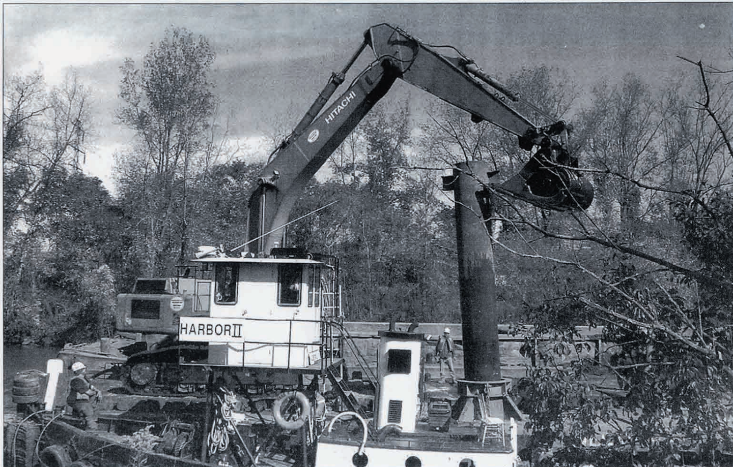
Spuds are lifted on one of the barges with a Rig-All Crane to adjust the barge's positioning.
